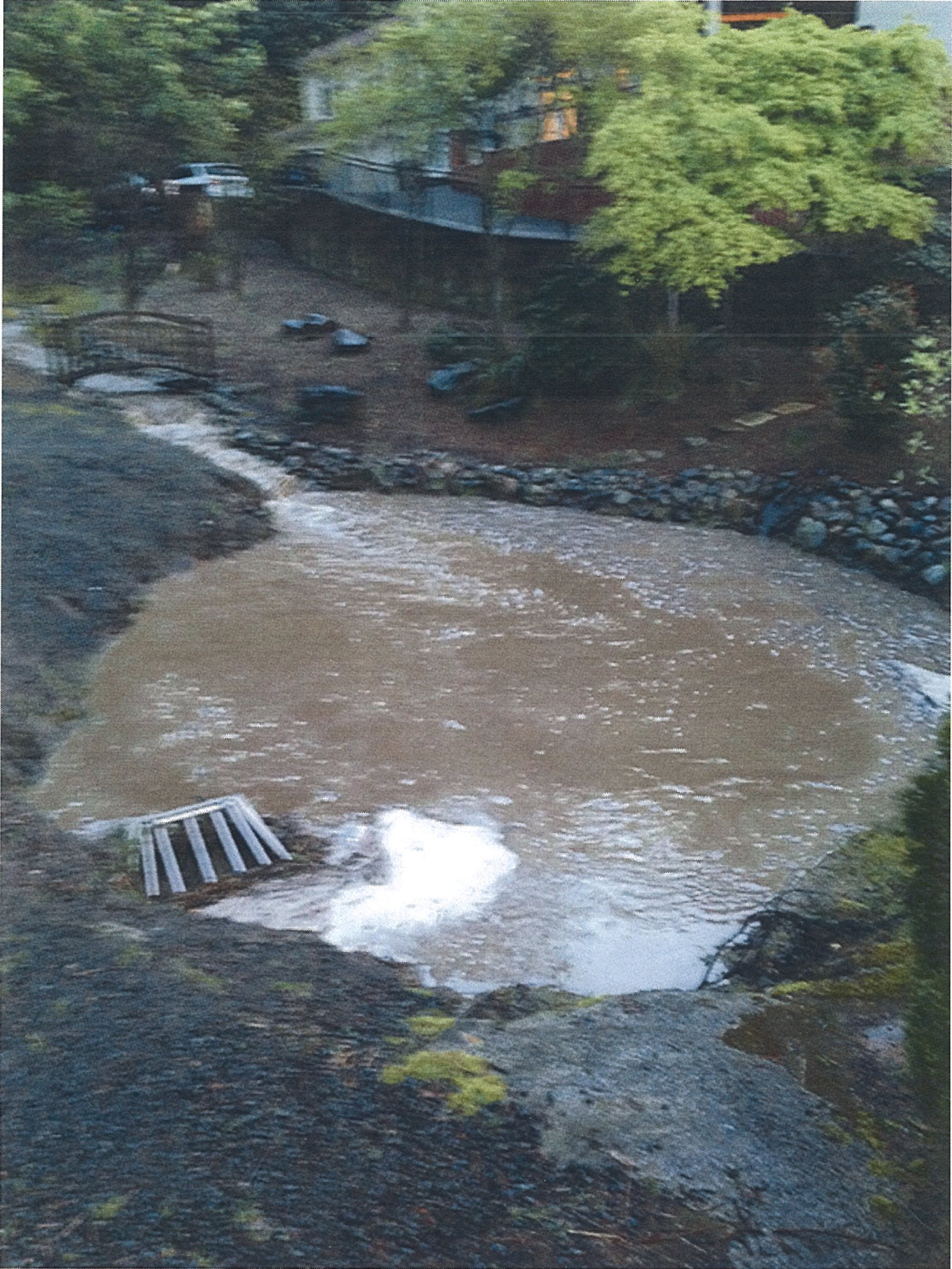
CITY MAINTAINED SILT POND Located at 5632 E. Mercer Way
